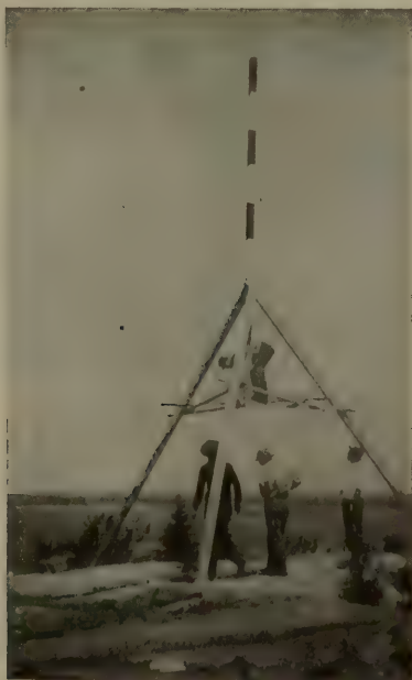
FIG. 11. Tripod Signal.
